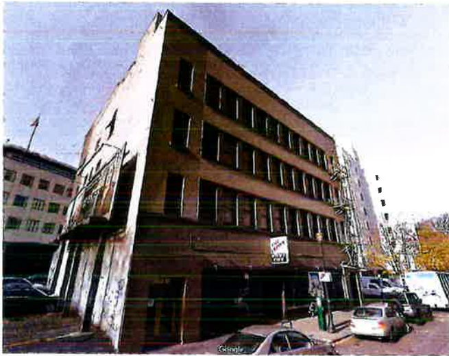
Existing Building View Looking Northwest on Park Avenue
